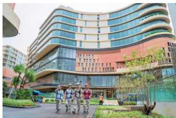
Tien Bo Plaza (Electrical equipment construction performed by Yurtec Group in Vietnam)
