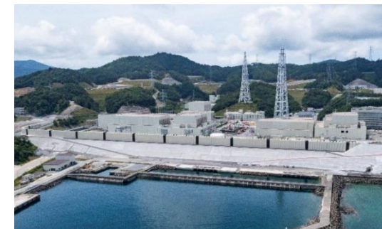
Onagawa Nuclear Power Station
