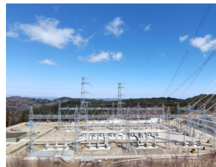
Miyagi Marumori Switching Station (500,000 volts) Installation status of new construction
