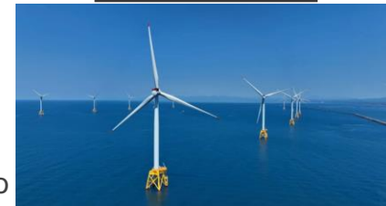
Ishikari-bay Shinko Offshore Wind Power Project (Photo courtesy of JERA)
