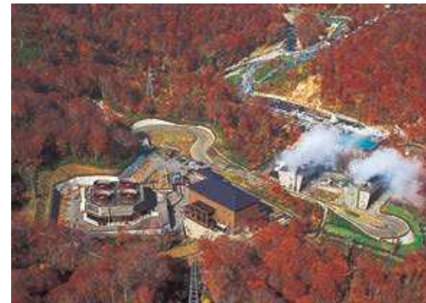
葛根田地熱発電所 Kakkonda Geothermal Power Station
