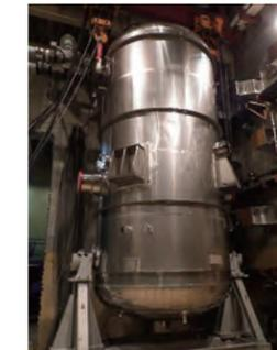
New venting equipment with filters for the containment vessel (Onagawa Nuclear Power Station)
