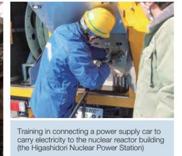
Training in connecting a power supply car to carry electricity to the nuclear reactor building (the Higashidori Nuclear Power Station)
