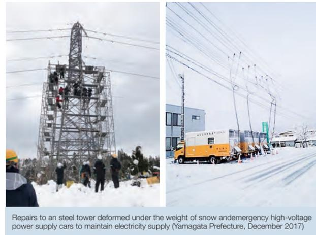
Repairs to a steel tower deformed under the weight of snow and emergency high-voltage power supply cars to maintain electricity supply (Yamagata Prefecture, December 2017)
