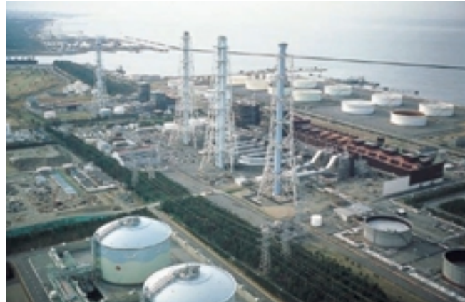
Higashi Niigata Thermal Power Station
