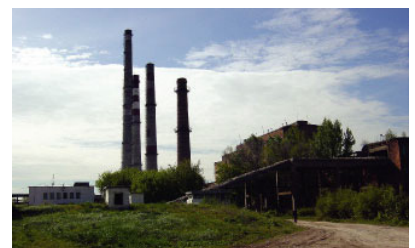
Uralsk Heat Power Station
