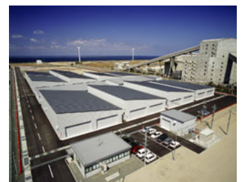
Sakata Storage Center
