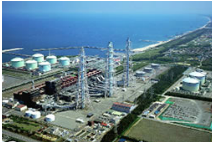
Higashi-Niigata Unit 4-1 System
