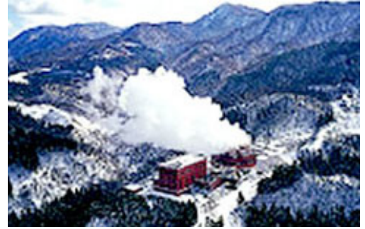
Yanaizu-Nishiyama Geothermal Power Station
