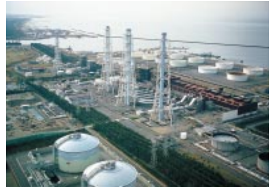
Higashi Niigata Thermal Power Station, Unit 4-1
