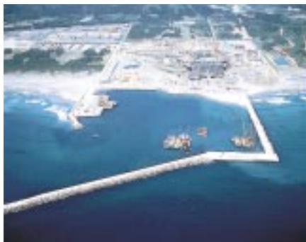
Higashidori Nuclear Power Station (under construction)
